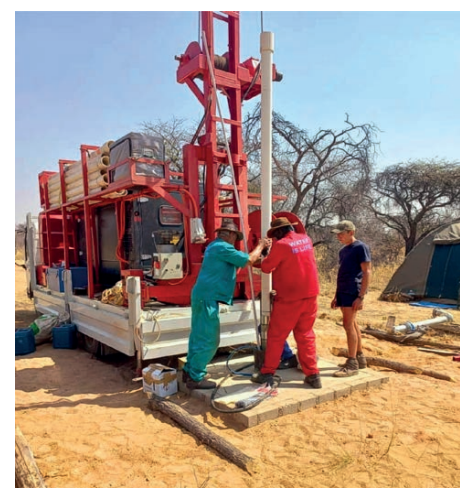
Foto: African Drilling
